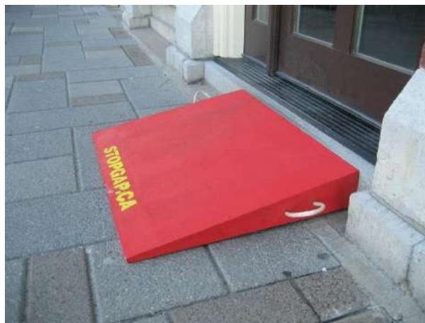
**Figure 21 - Customized portable ramps are a simple method to improve accessibility**
