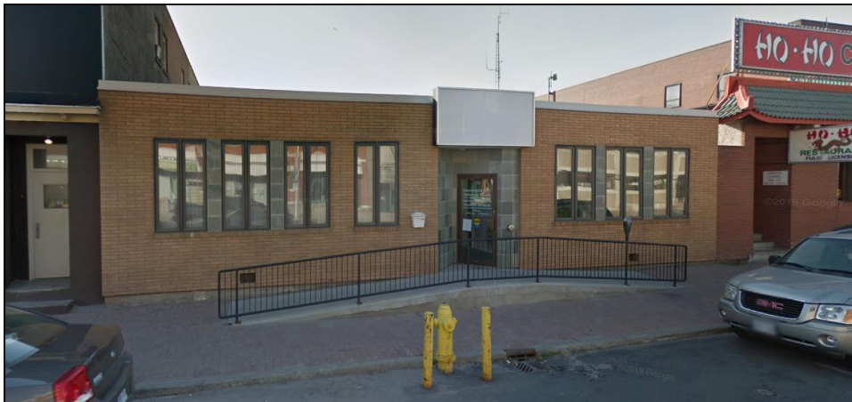
Figure 4-3: Kenora District Services Board Building with wheelchair access ramp, 120 Matheson Street South, Kenora, ON (Source: Google Streetview, 2022)
