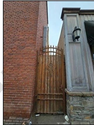
Figure 4-4: Example of security gates at recessed and central doorways and laneways within Harbourn Centre (Source: City of Kenora)
